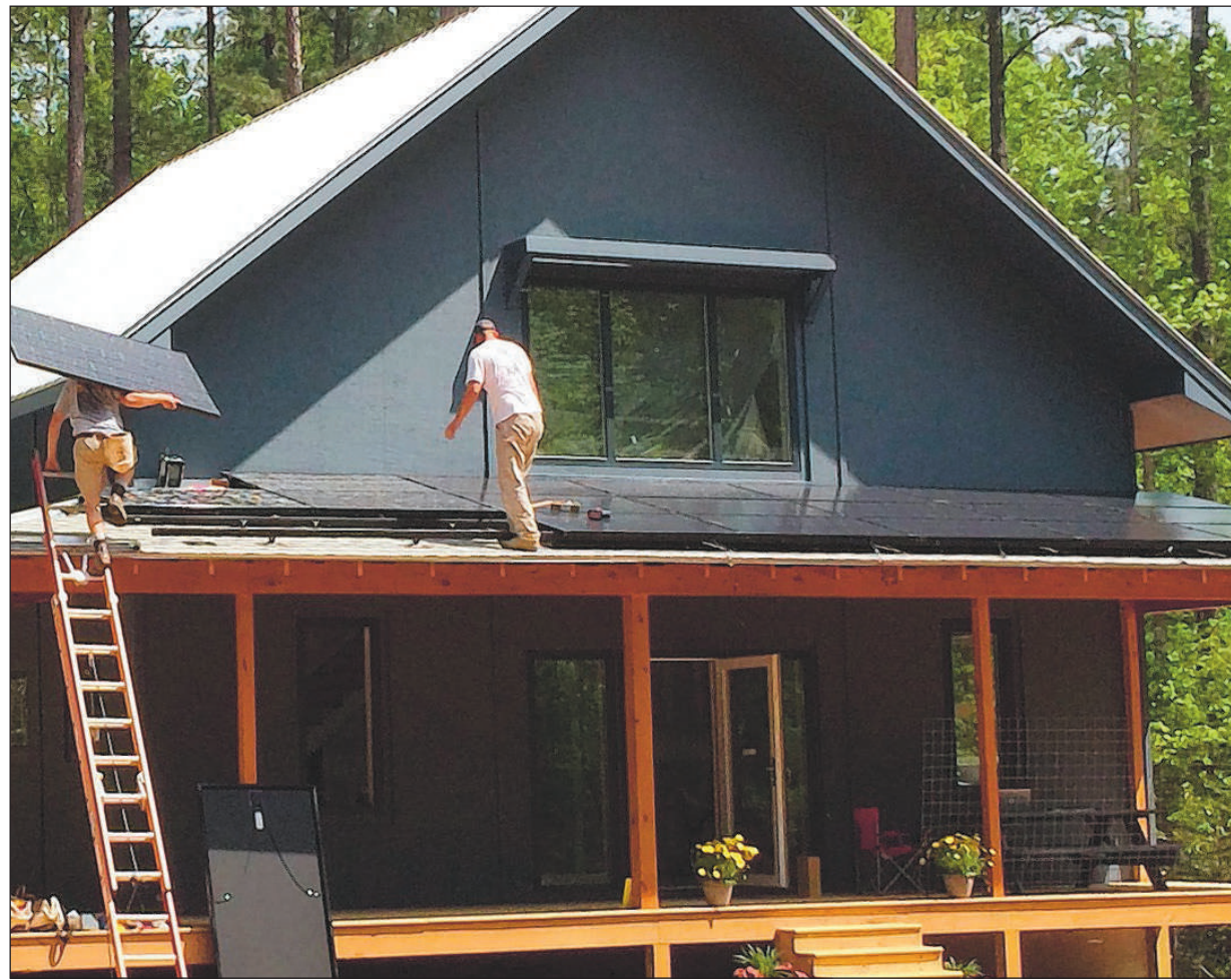
PHOTOS BY SALLY KEENEY Twenty 3- x 5-foot solar voltaic panels will run all the electrical, including washer, dryer, all electric lights and whole-house heat using an LG mini-split HVAC. This net-zero-energy PassivHaus, built by Anchorage Building Corporation's Chris Senior and Joe Norwood, has a propane tankless hot water heater.
